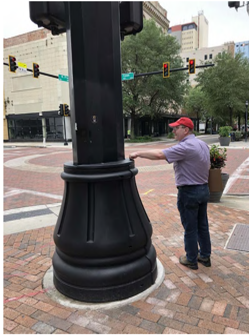
Oversized mast arm bases
