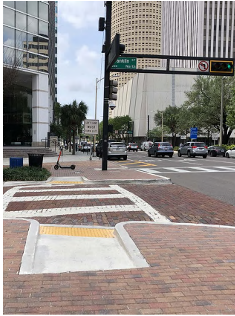
Crosswalk and narrow ramps
