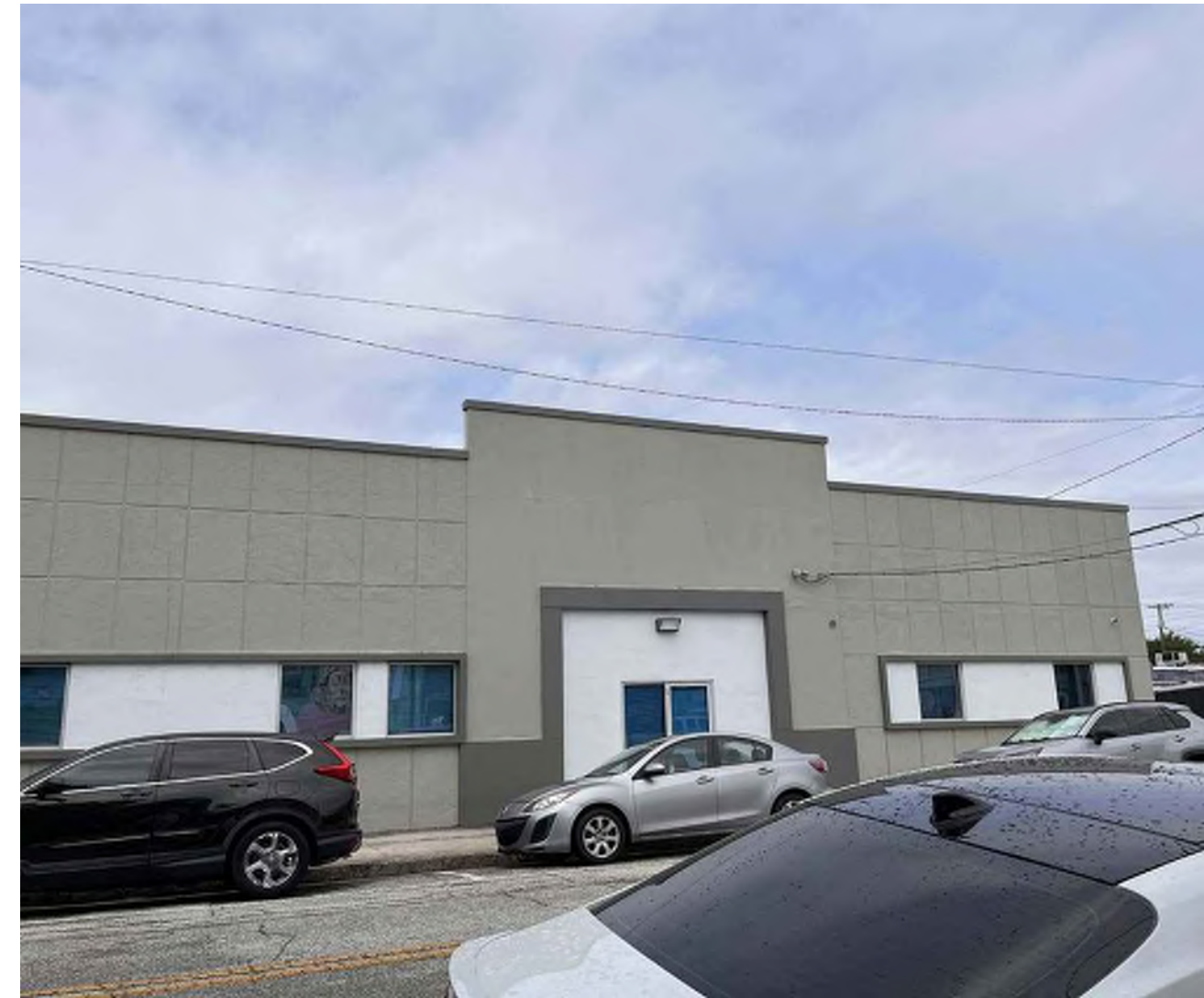
Blank facade along streetscape
