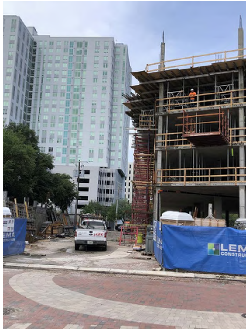
New hotel property under construction
