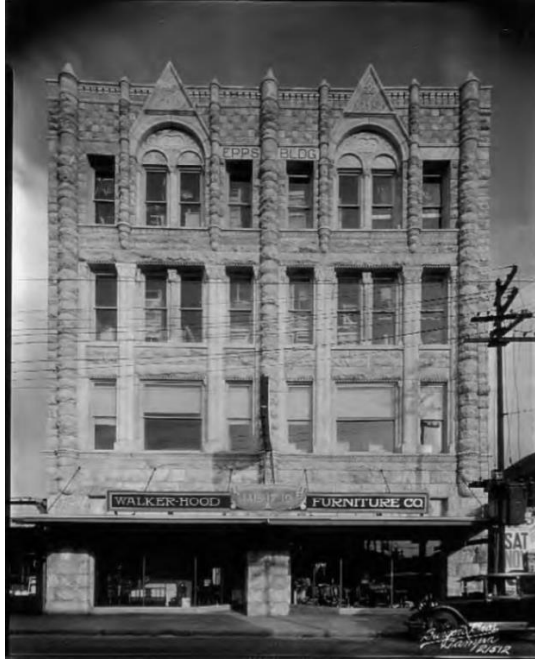
Eps Building (1415-1417 Franklin St)
