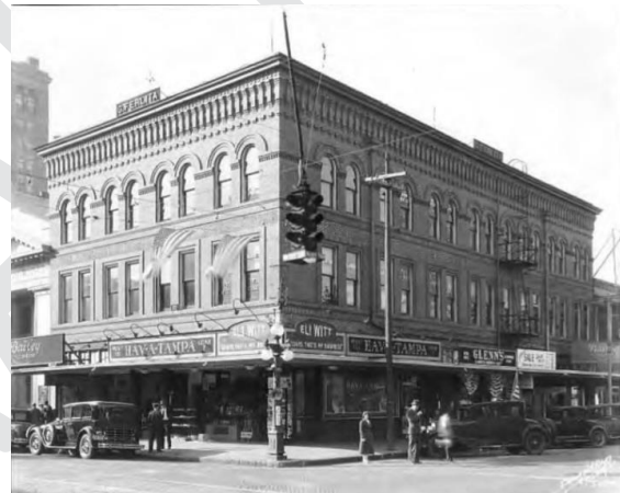
Ferlita Building (corner of Twiggs and Franklin St)
