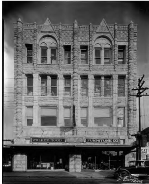
Eps Building (1415-1417 Franklin St)
