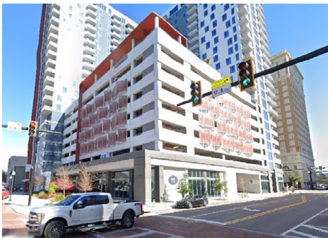
East Cass St./North Franklin St. (before and after)
