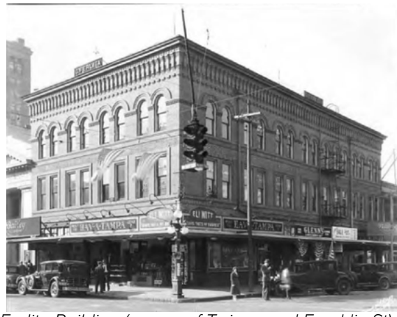
Ferlita Building (corner of Twiggs and Franklin St)
